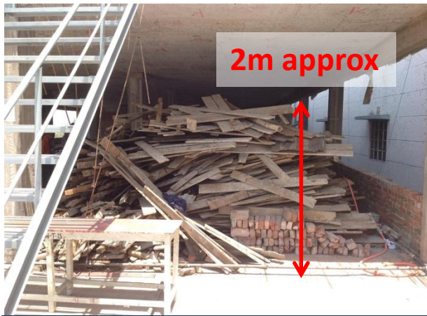
Construction storage on slab associated with ongoing construction at roof level.
