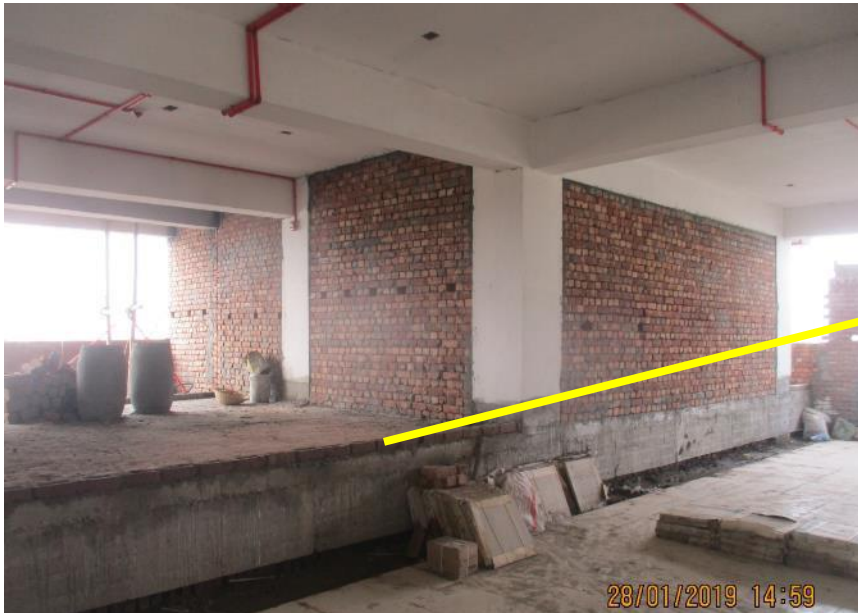
Different slab height on 1 st floor
