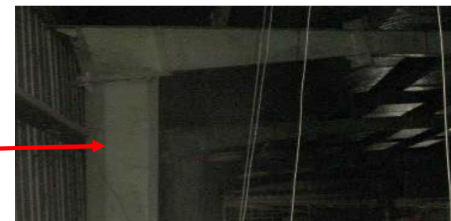
Uniformed section was found instead of tapered section
