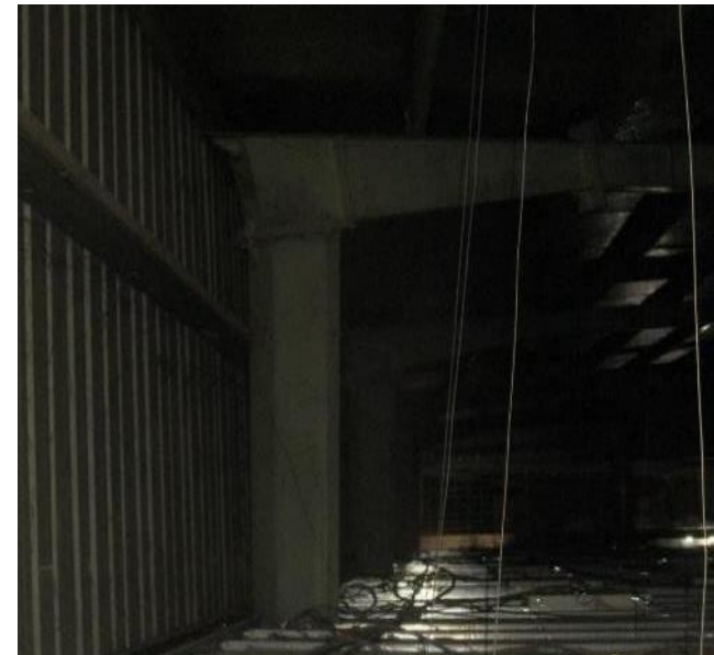
Steel frame (No vertical bracing)
