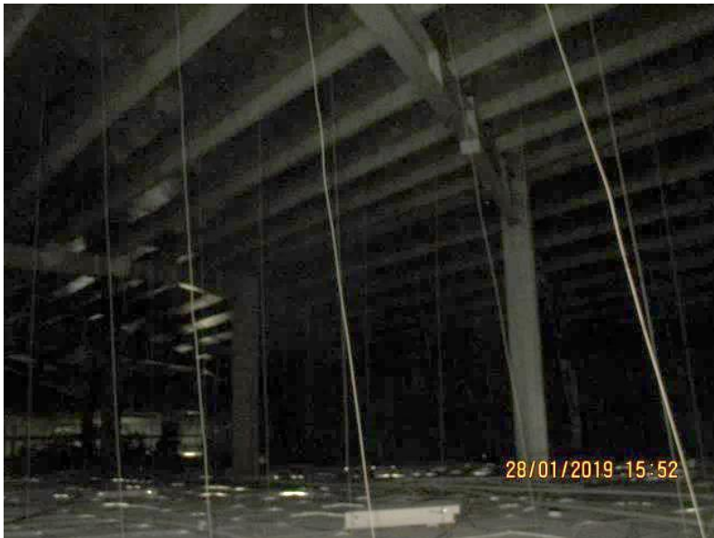
Steel frame (No Roof/Horizontal bracing)
