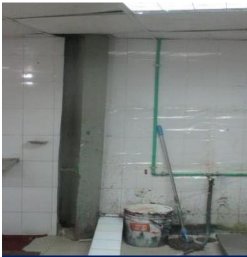
Steel columns were bolted
