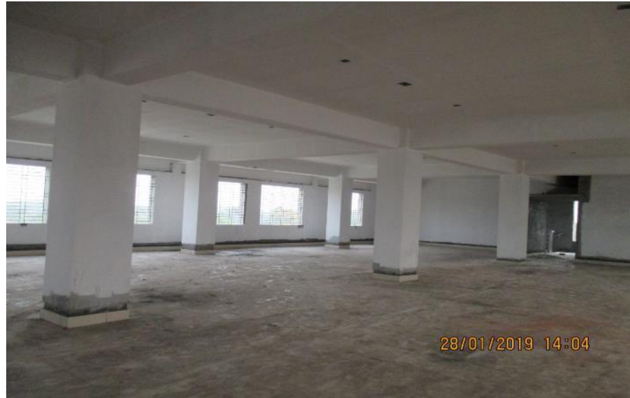
Unoccupied 4 th floor
